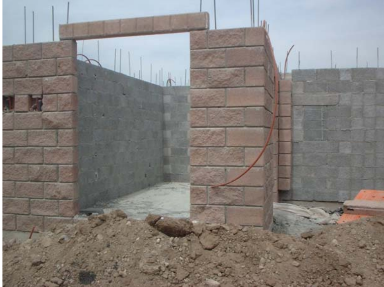
Figure 5 Most of houses in Mexico are made of brick or block
