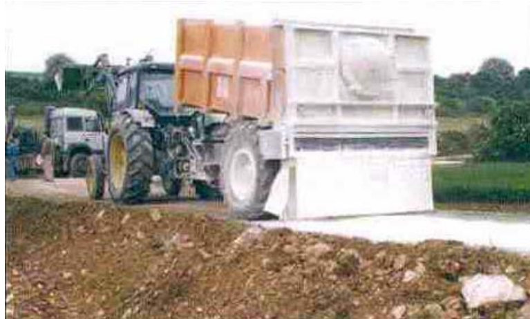
Figure 4 Soil stabilization using bulk lime
