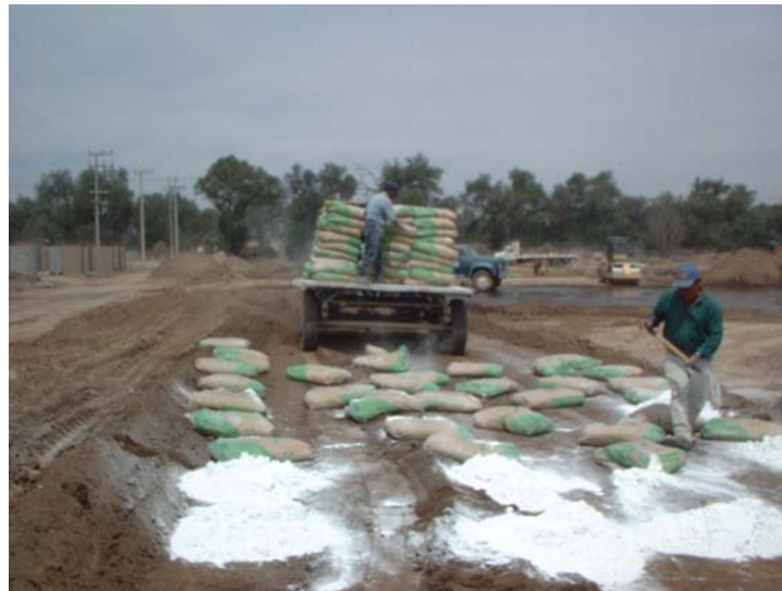
Figure 3 Example of bag use in lime stabilization
