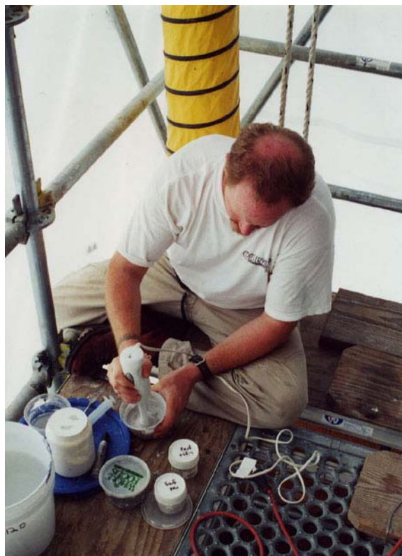
Figure 4: On-site mixing of DHL for injection.
