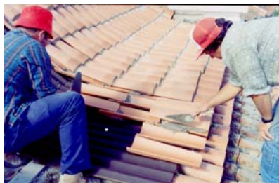
Figure 8—Ceramic tiles placed over a synthetic under-roof
