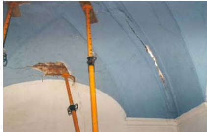
Figure 7- Detail in interior of the vestry vault
