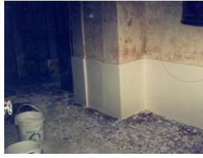
Figure 15- New plaster made with lime putty mortar with marble dust
