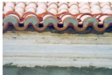
Figure 9- Detail of the roof edge finishing
