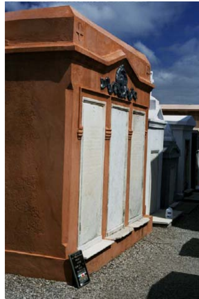
Figures 3 and 4. The Malard Family tomb, before and after restoration. Work on this tomb included significant re-stuccoing, repair of marble closure tablets, recreation of missing metal decoration and application of its historic colored limewash (photographs by author).
