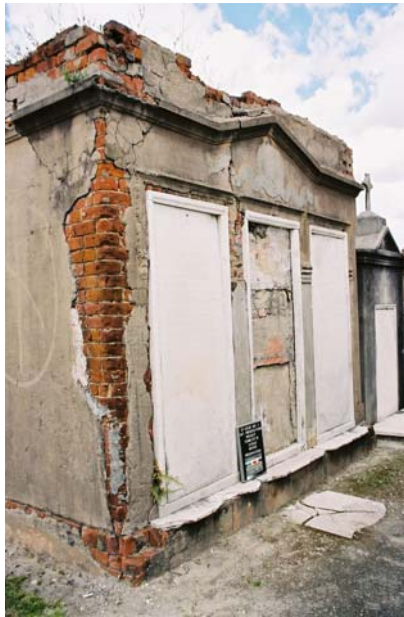
Figures 3 and 4. The Malard Family tomb, before and after restoration. Work on this tomb included significant re-stuccoing, repair of marble closure tablets, recreation of missing metal decoration and application of its historic colored limewash (photographs by author).
