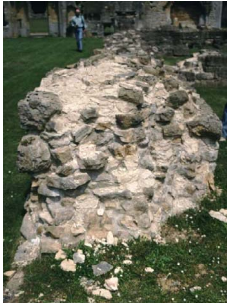
Figure 1. An example of the capping of a ruin wall.
