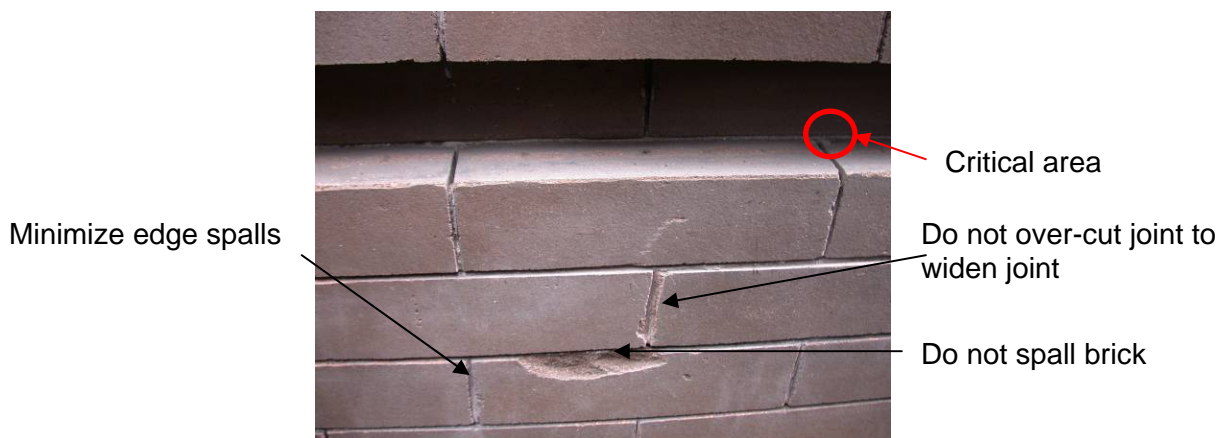
Figure 5 Sample of instructions from joint preparation guide
