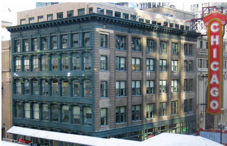
Figure 1 View of north and west facades of building.
