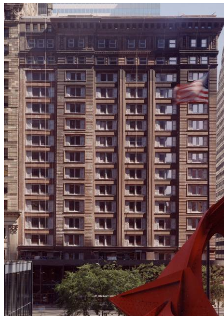
Figure 4 Overall view of south facade
