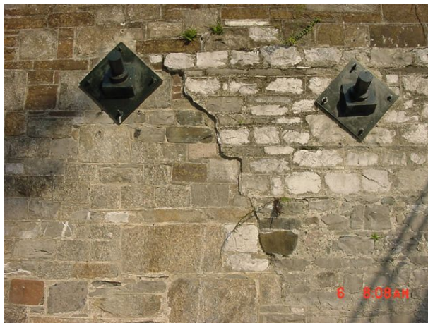
Figure 8. Cracks in Historic masonry retaining walls on Factors Walk, Savannah, GA, before and after injection with a combination of fine and coarser polymer-modified grouts.
