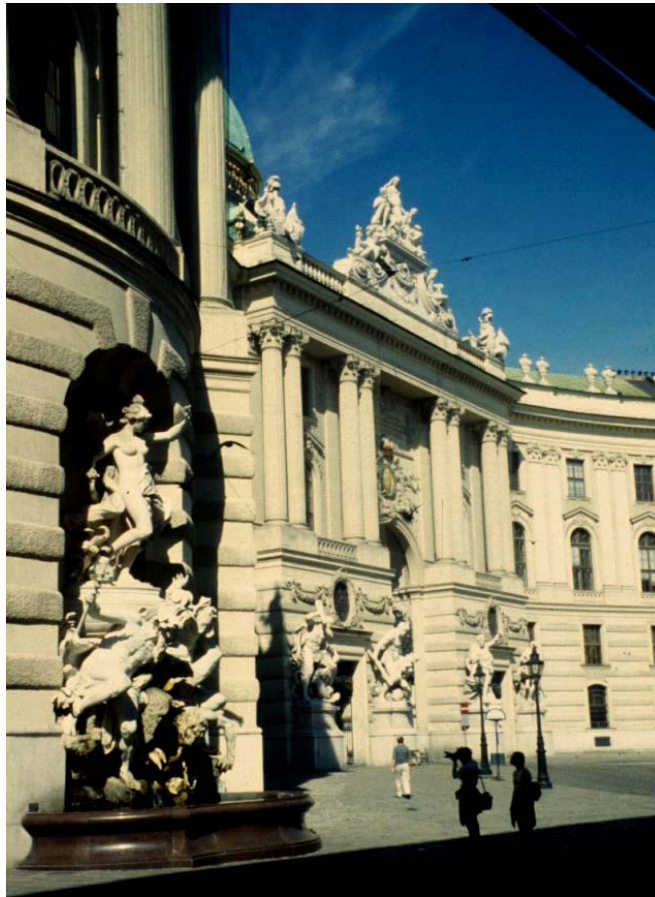
Figure 2 View of the entrance to the Hofburg in Vienna (Austria). The sculpture group that decorates one of the two fountains is carved of Laaser marble (seen at left), while the other sculpture groups are carved in a soft limestone and have received a lime-based sacrificial coating.
