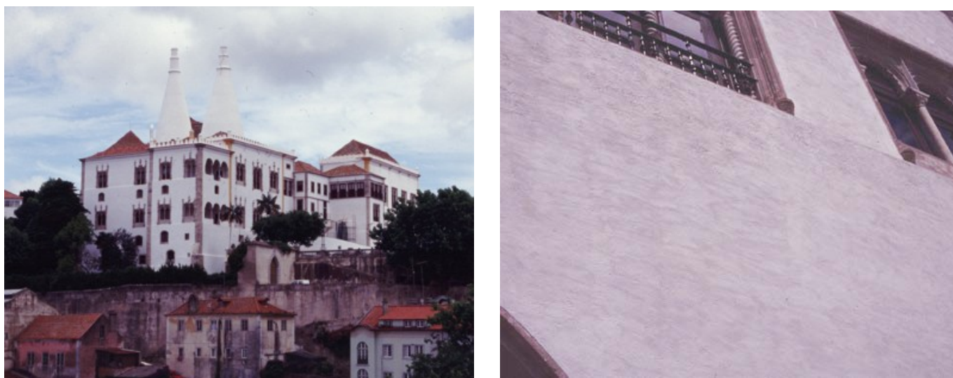
Figure 3 The large conical chimneys at the National Palace of Sintra are its landmark feature (left). Detail of the final appearance of the cleaned and patched render (right). The traditional lime formulation showed excellent compatibility with the original render.
